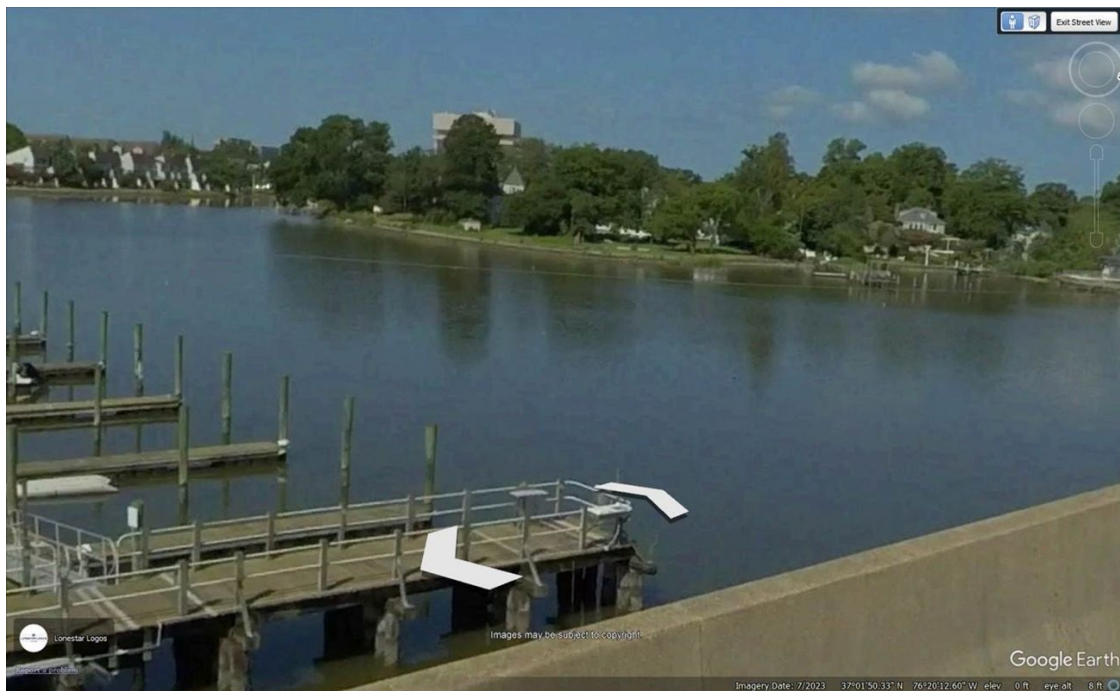
Figure 1. Google Earth Street View, imagery date July 2023 (GE1), taken from the old eastbound bridge sidewalk at 37°01'50.33"N, 76°20'12.60"W. The end platform is intact: pipe rail and posts straight, pile caps seated, diagonal cross-bracing in place under the deck, floating docks level, no barges. Independent third-party evidence of pre-construction condition, and of how close the platform sits to the bridge.
