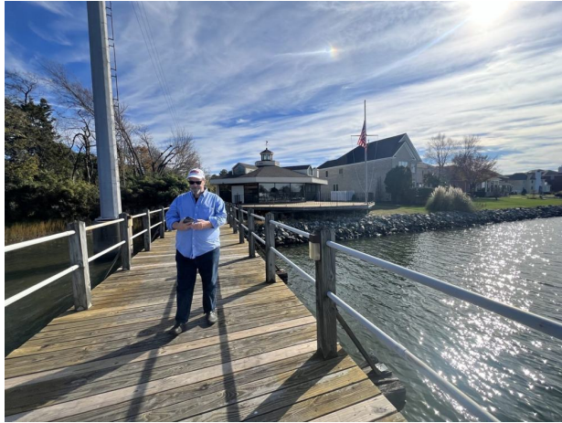
Figure 2. Baseline, November 20, 2023 (A03, A04). Deck line level, rails straight, the diagonal pile-to-post tie at the right-hand rail post fully seated; slips full; no barges or cranes near the pier.
