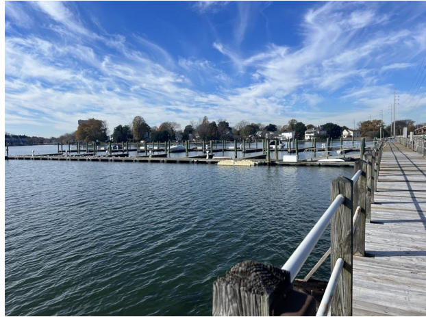
Figure 2. Baseline, November 20, 2023 (A03, A04). Deck line level, rails straight, the diagonal pile-to-post tie at the right-hand rail post fully seated; slips full; no barges or cranes near the pier.
