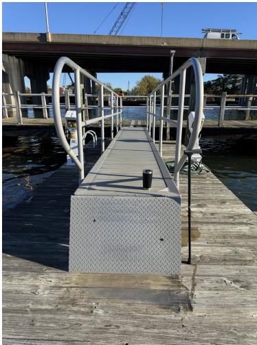
Figure 3. Baseline, November 16, 2024 (B01, B02). Gangway and float landing level; guide piles and floating docks square. A crane boom is visible above the old bridge, consistent with the westbound widening then under way.
